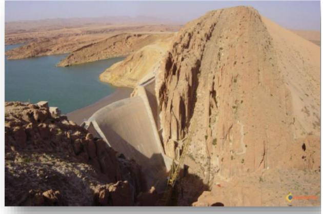
Figure 1: Brezina concrete arch dam [ref. Wikipedia.org]
